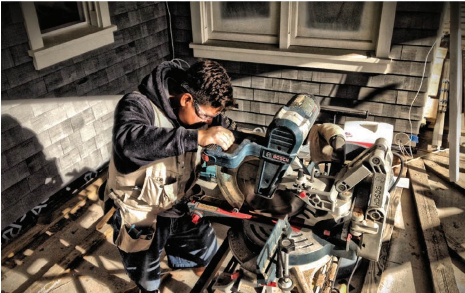
Photograph by Rick Carrillo, Lead Carpenter at Millworks by Design
