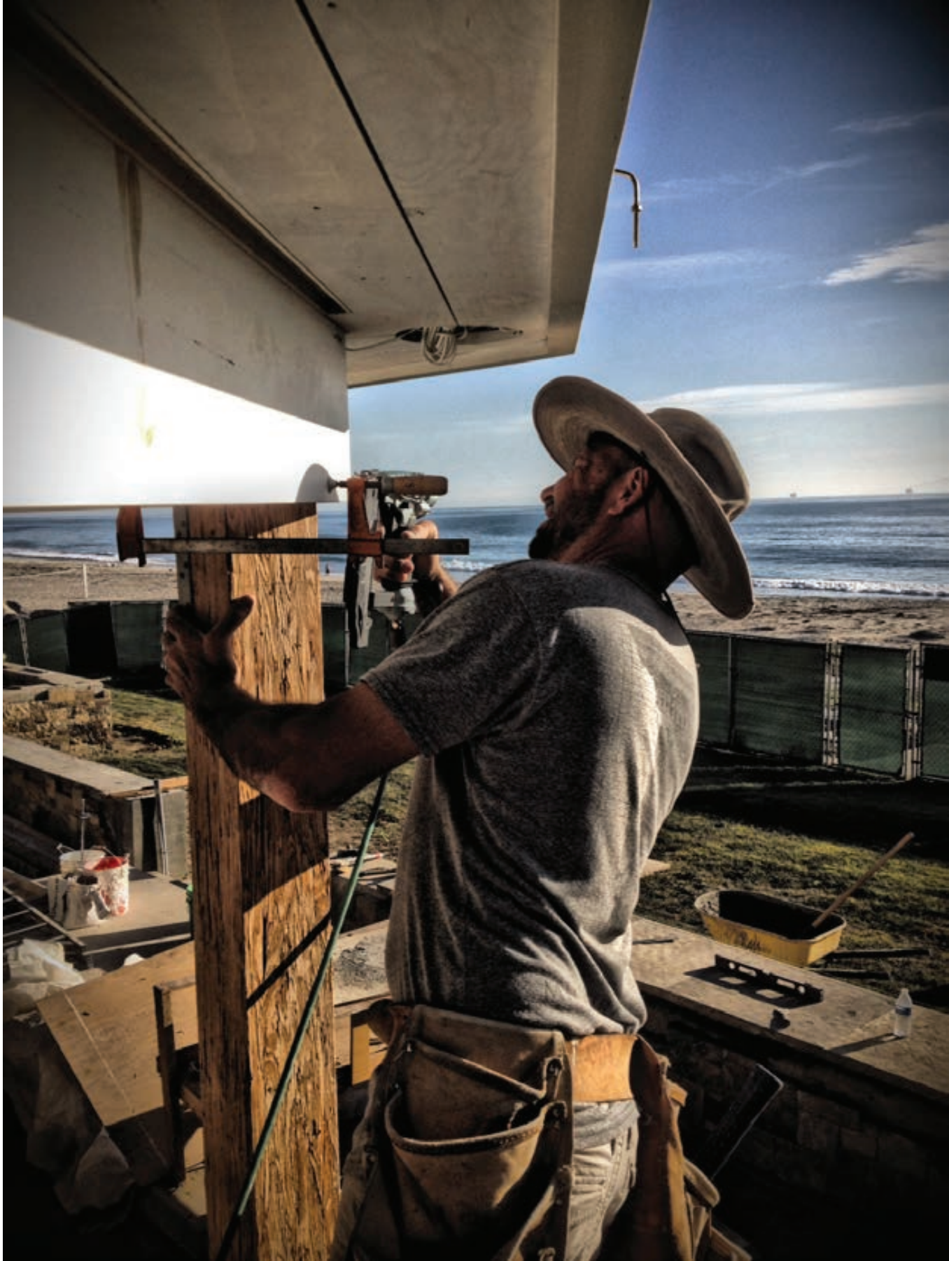
Photograph by Rick Carrillo, Lead Carpenter at Millworks by Design
